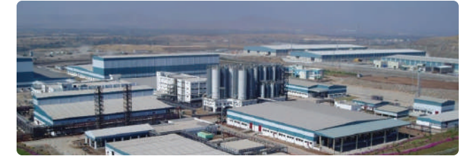
Aerial view of Khandala plant
